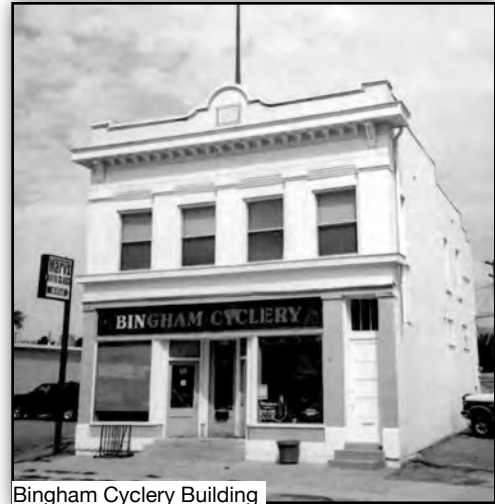
Bingham Cyclery Building
